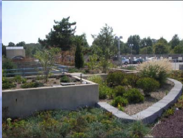
Green roof: Herry parking structure
